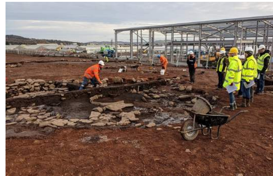
Excavation prior to development at the Hutton Institute, Invergowrie.
