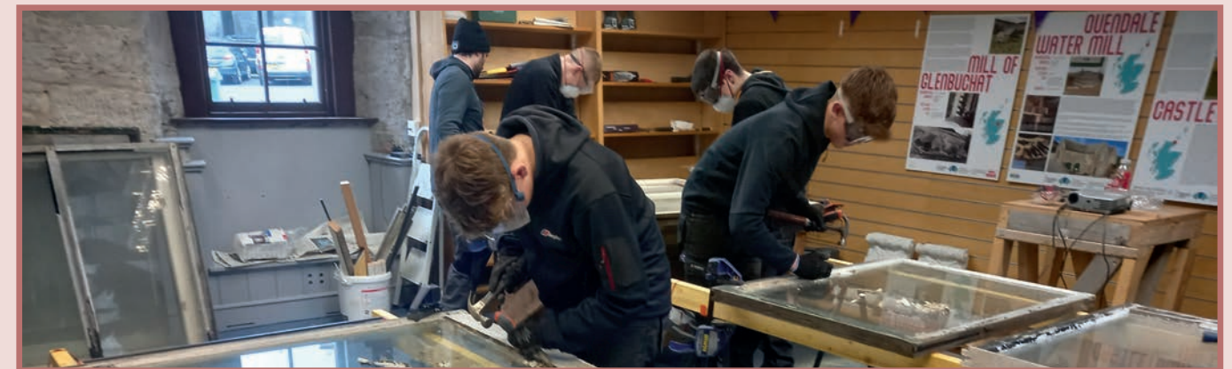
Mosaic Restoration students at assemble piece prior to installation at the City Mills, and young people learn about refurbishment of sash and case windows.
