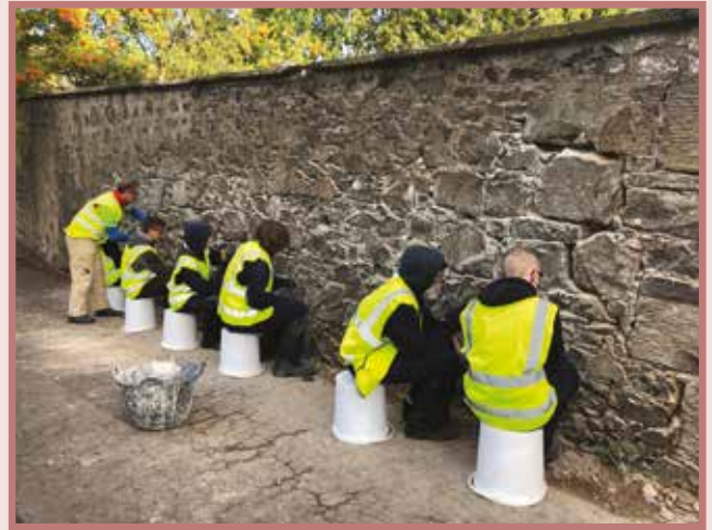
St John's Academy pupils and trainer racking out cement mortar at Murray Royal Walled Garden, Perth (photo: Craig Frew).
