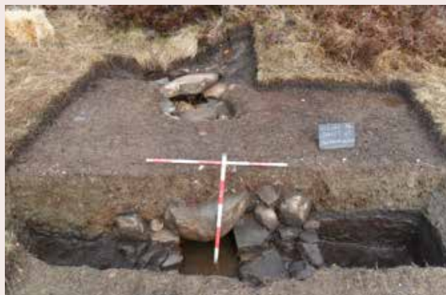
General Wade road culvert near Amulree uncovered during work on the Beaully to Denny electrical power-line. (courtesy of Northlight Heritage & SSE)
