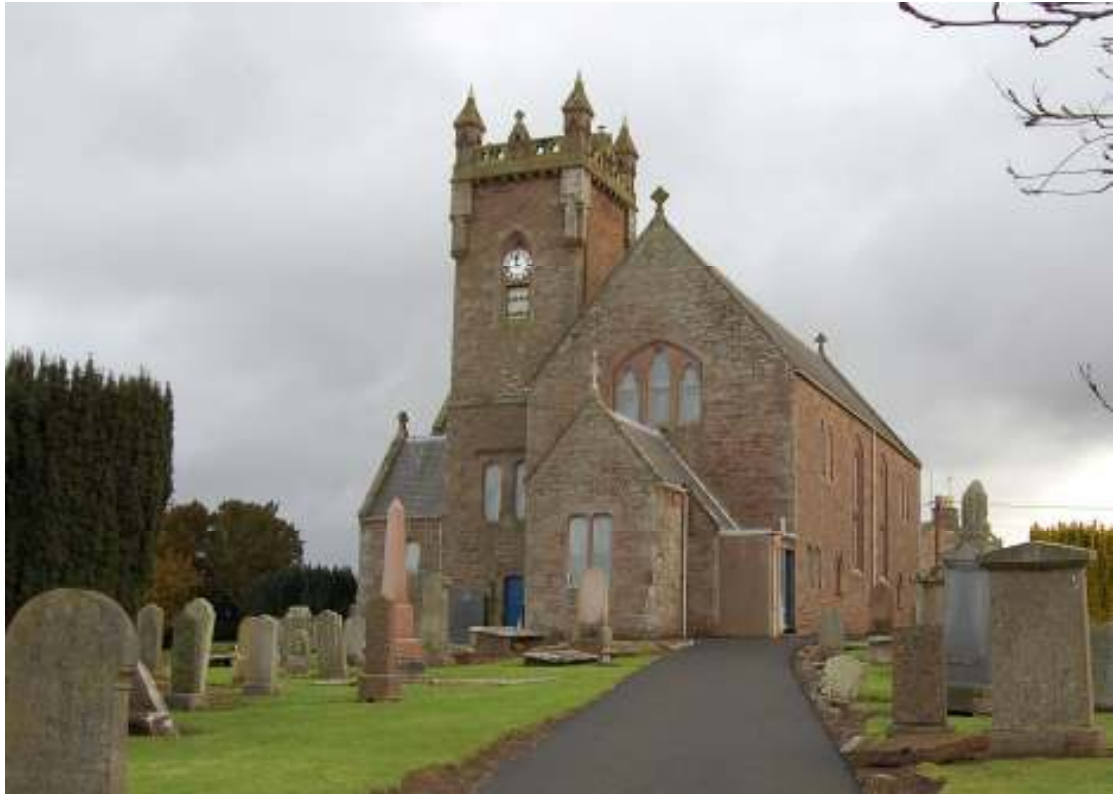
Meigle Parish Church, March 2011
