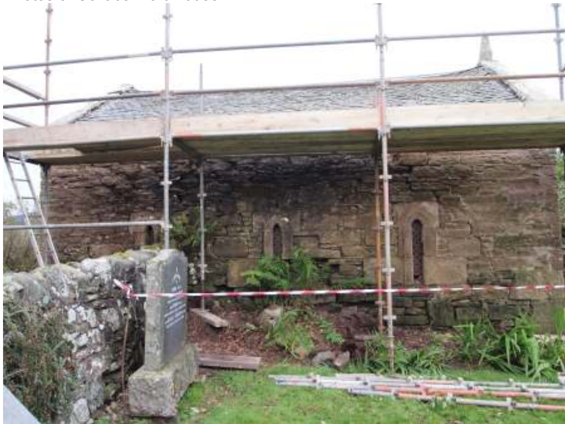
Mort house under repair
